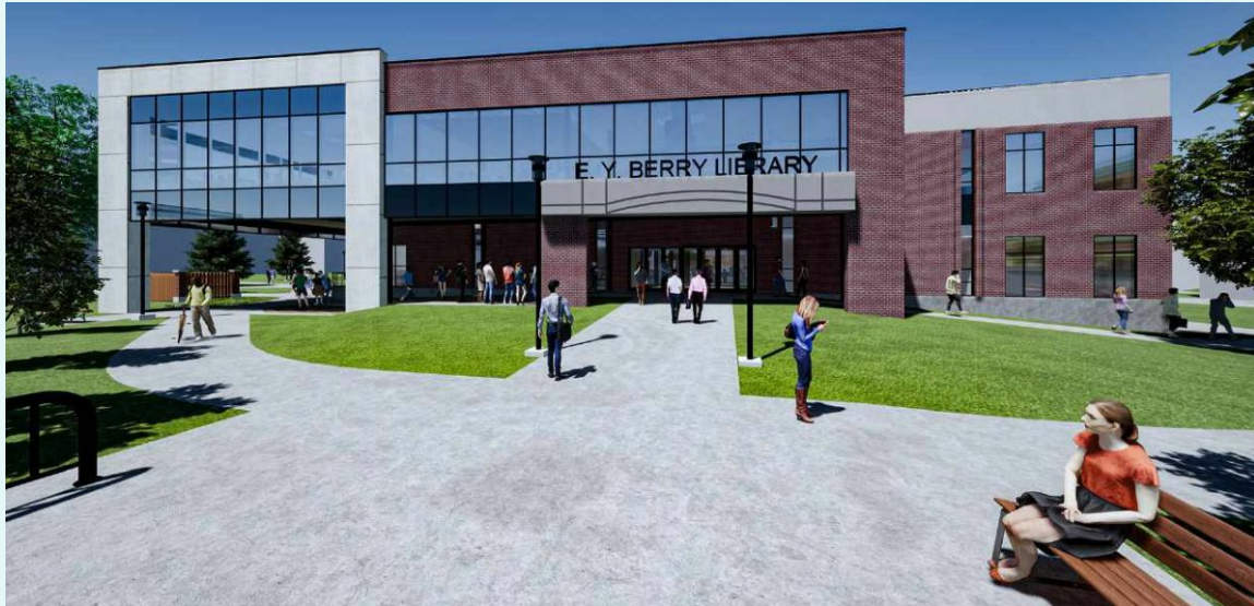
Design of the in-progress Black Hills State University Library Renovation
